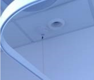
Original ceiling mounted cords
