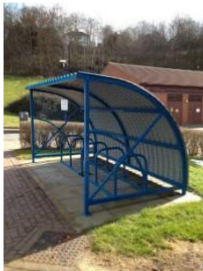
Figure 2.5 – Cycle stands close to the building entrance
